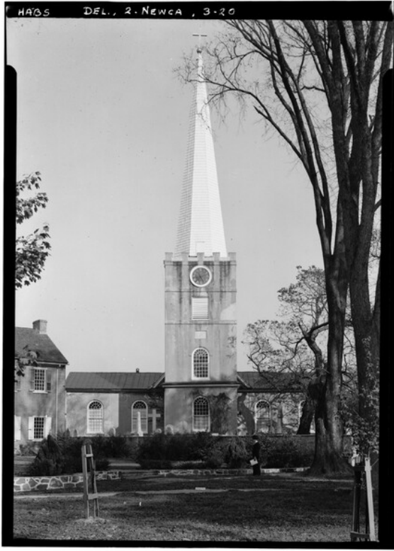
fig. 1 W. S. Stewart, West Facade—Immanuel Church (Episcopal), The Green, New Castle, New Castle County, DE , October 23, 1936, photograph, Library of Congress, Prints and Photographs Division, Washington, DC
